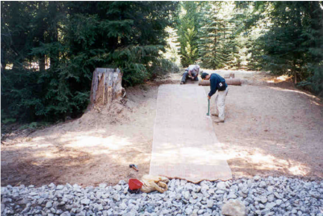
Above: LAYING GROUND MATS FOR EROSION PROTECTION
